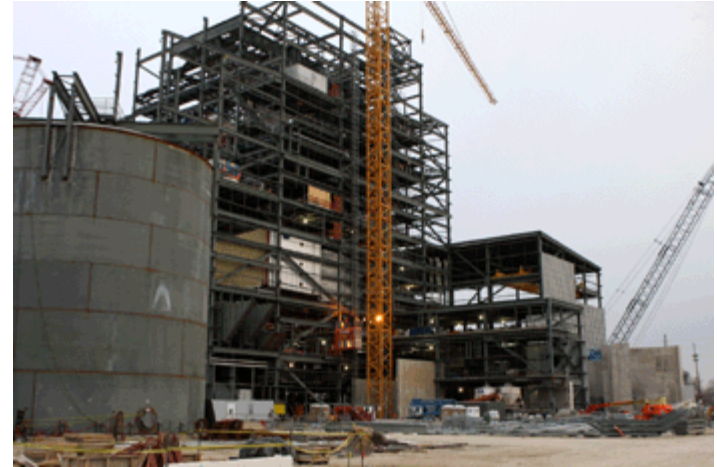
Construction of new coal power plant in Illinois (source: www.cwlp.com )
