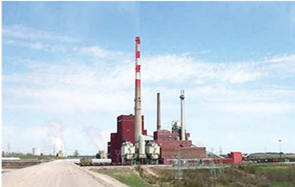
1. Stable response. A new boiler master design improved the stability and response of Unit 3 of E.ON U.S.'s E. W. Brown Generating Station. Courtesy: E.ON U.S.
