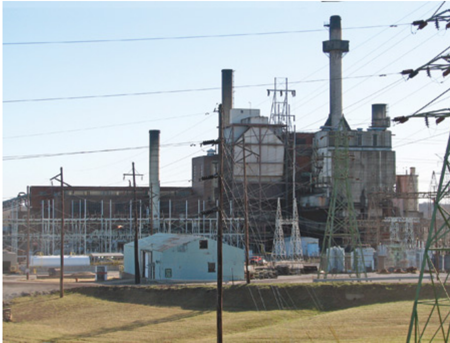
3. Twin projects. Significant heat rate reductions were the result of boiler master updates at E.ON U.S.'s Green River Generating Station. Courtesy: E.ON U.S.
