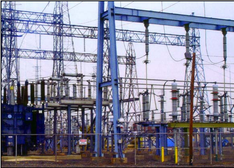
Essex Switching Station Modification of towers and connections
