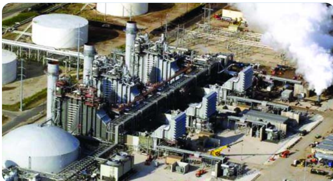
Burns and Roe provided engineering, procurement and startup support services the Texas City CHP Project, a 650 MW combined cycle cogeneration plant in Texas.
