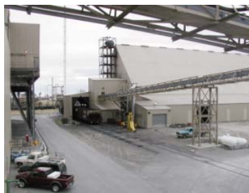
Yellowstone Energy Project Billings, Montana
