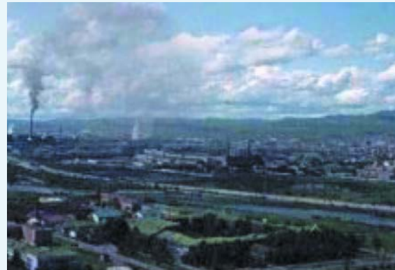
Ulaanbaatar, Mongolia - The central heating plant is the only source of heat and hot water in the city.
