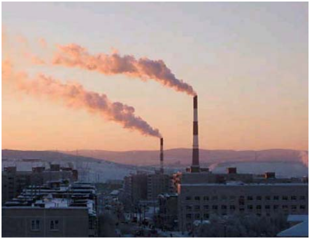
Murmansk, Russia - Burns and Roe directed the rehabilitation of the Central Heating Plant.
