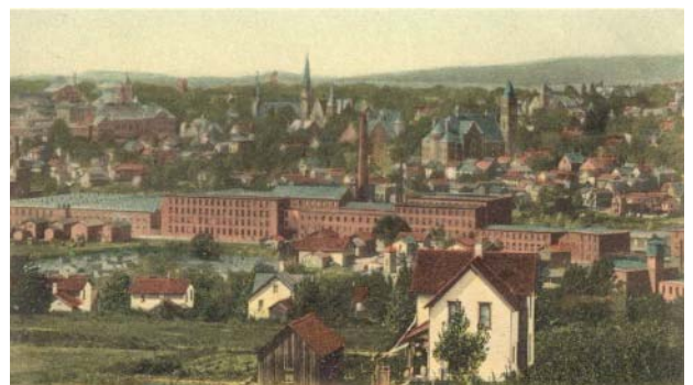
City of Jamestown - Burns and Roe designed, installed, and later expanded the original District Heating System.
