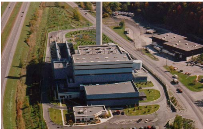
Onondaga Resource Recovery Facility 40 MW/990 TPD - Solid Waste to Energy Facility, Onondaga, NY
