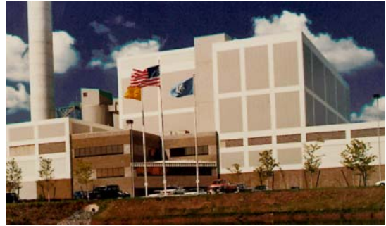
Bristol Resource Recovery Facility 13 MW/650 TPD - Solid Waste to Energy
