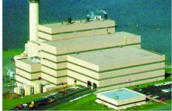
Westchester RESCO Refuse-to-Energy Facility 2250 TPD/60 MW - Waste to Energy Facility, Peekskill, NY
